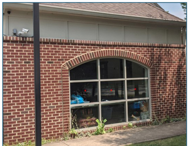
A Nonprofit Security Grant was used to install security cameras and forced entry-resistant windows at this location in Wilmington.
